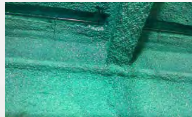
ABC Green applied to asbestos containing fireproofing on structural steel beams
